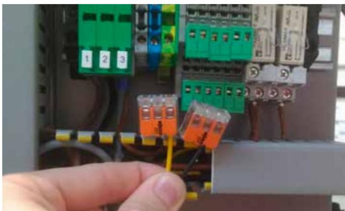
Tipo cavo MODBUS: Templari HCC cable (tipo Belden 3105A 2x22AWG shielded)
